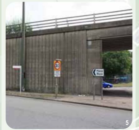
Poor wayfinding and signage throughout Manor Royal
