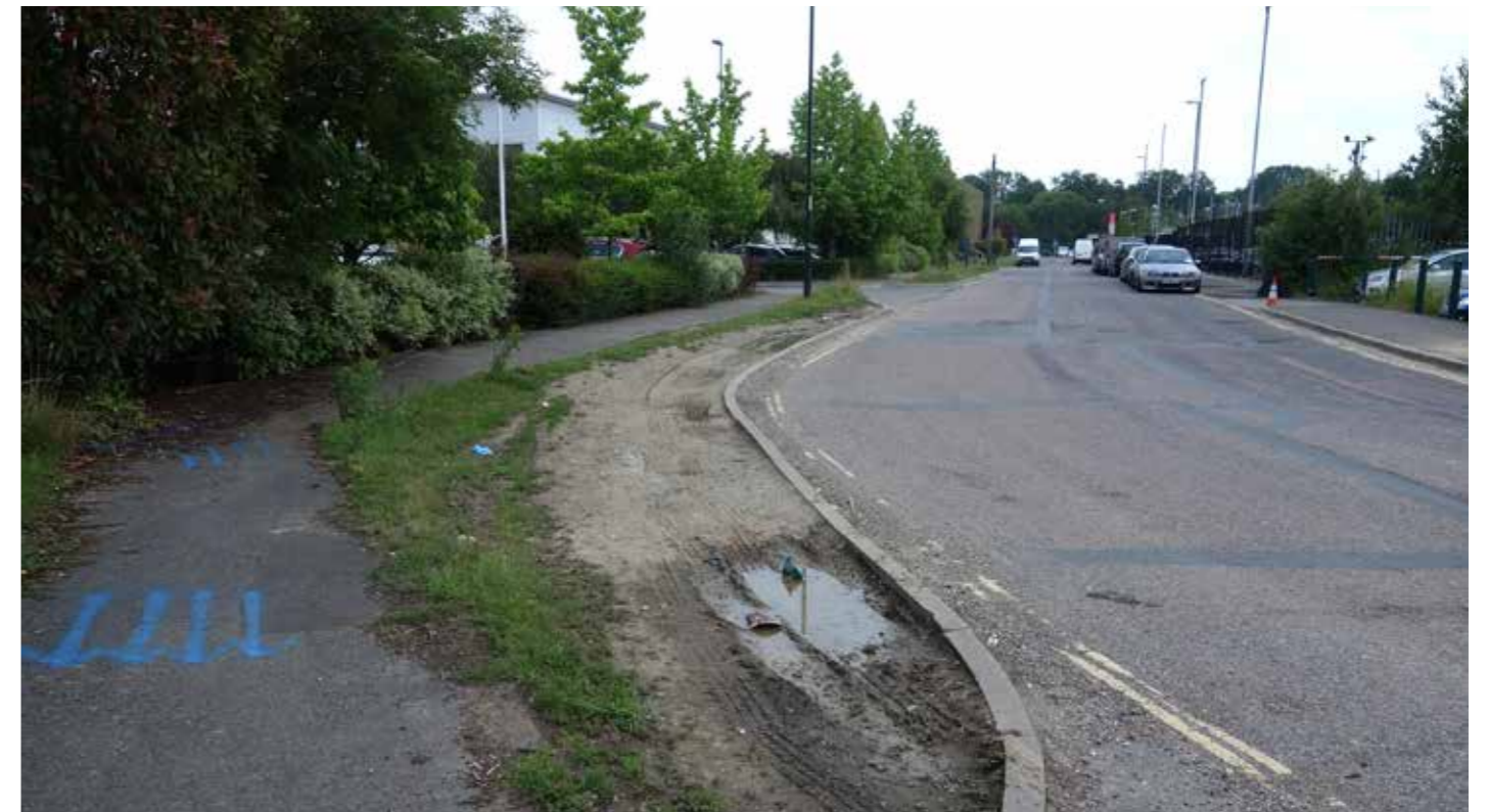
Grass verges on Napier Way suffer from constant pounding from trucks and cars.
